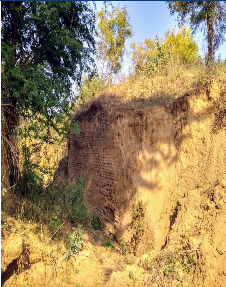
Figure :21 Exposed brick wall
