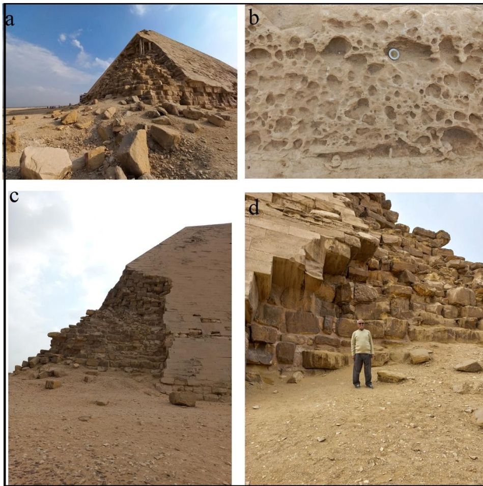
Fig.5: Effect of weathering process on the stones of The Bent Pyramid (a: The effect of weathering processes on the breakdown of rock masses in the northwestern corner of the pyramid; b: The effect of chemical weathering processes by water vapor on one of the rock masses on the northern side of the pyramid; c: The effect of weathering processes on the collapse of the northwest corner of the pyramid; d: The effect of weathering processes on the breakdown of the lower part of the stones of the pyramid)
